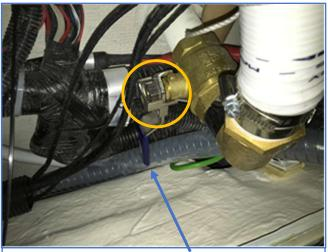
Waste discharge Seacock handle (closed here)
