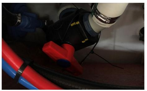
Valve closed, perpendicular to the line
